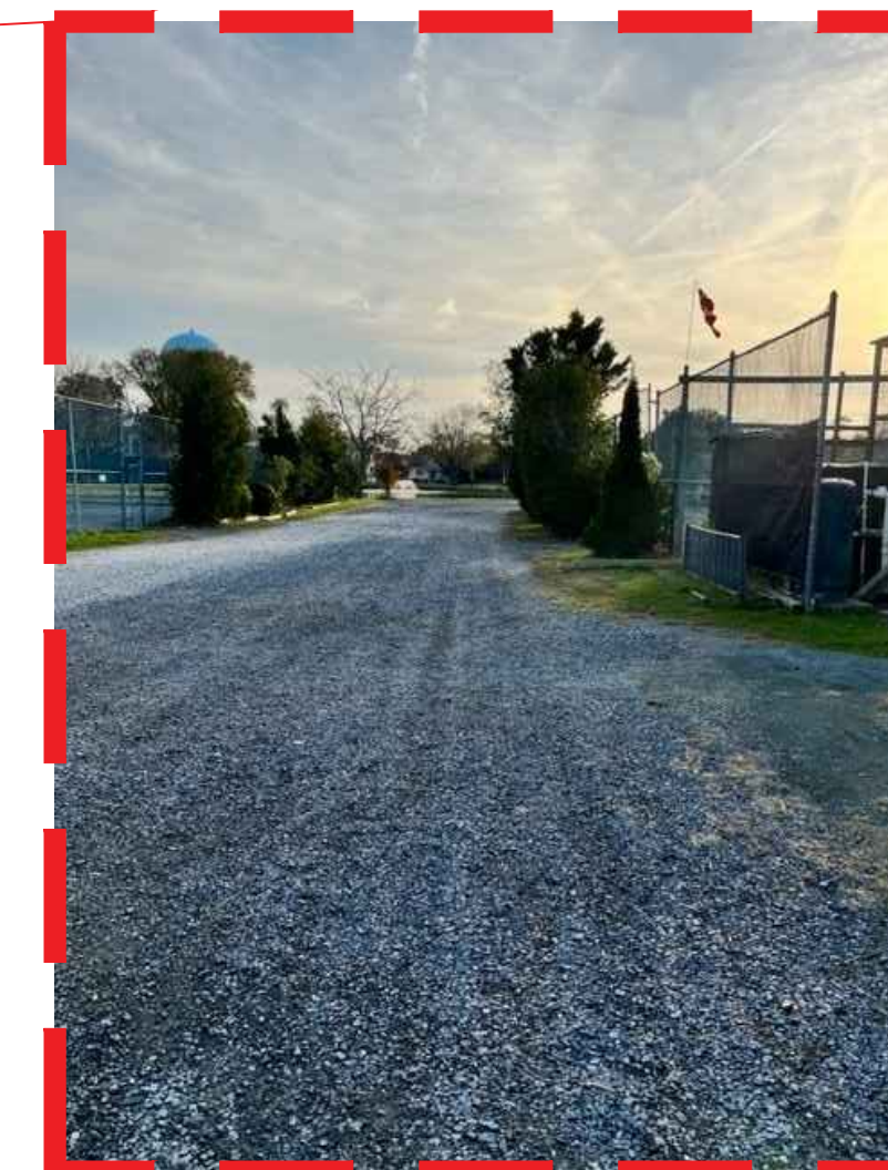
EXISTING ADA TENNIS COURTS CONSTRUCT CROSS WALK AND HANDICAP PARKING SPACE AT ADA ACCESSIBLE TENNIS COURTS
